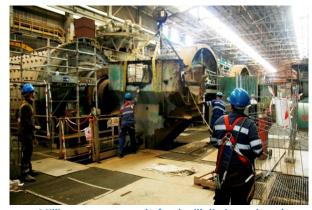
Milling area - removal of rod mill discharge launder
