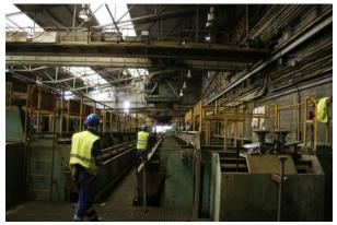
Flotation area - cells agitators dismantled and sent to workshop
