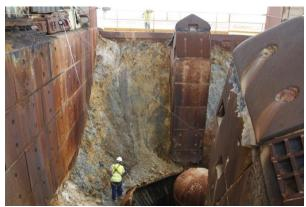
Crushing area — clean-up of primary crusher feed hopper
