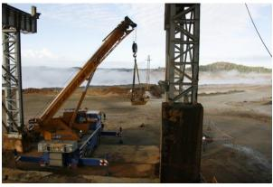
Crushing area – replacement of primary apron feeder sections
